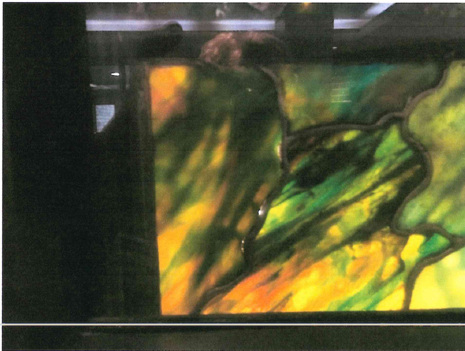
Clean and fill small daylight areas
